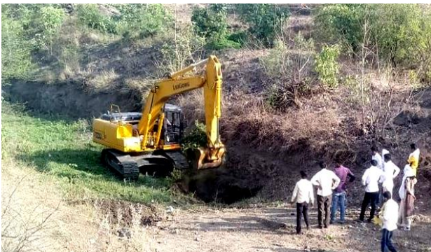
Canal deepening/desiltation
